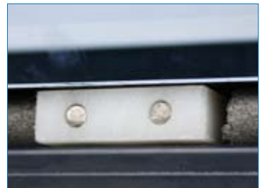
Load transferring packer (Petschenig)
