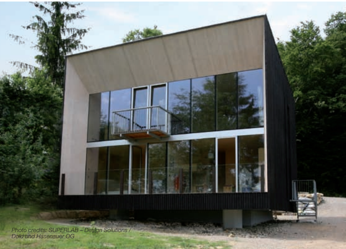
THE OTTO BUILDING WITH TIMBER-GLASS-COMPOSITE UNITS
