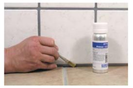
3. Possibly prime the adhesive flanks with the appropriate **OTTO Primer or Cleanprimer** with a soft paintbrush on absorbent substrates or with a soft cloth on non-absorbent substrates.
