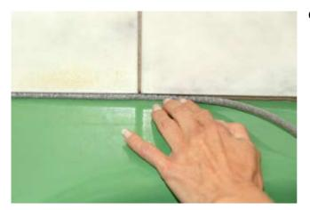
6. Back-filling of the cavity by inserting the appropriate OTTOCORD PE-B2 backer rod.
