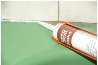
**3.** Apply a thick layer of **OTTOSEAL® SilOut** to the area to be treated - at least 5mm. After the **OTTOSEAL® SilOut** has taken effect, remove the dissolved silicone masswith a spatula and a damp cloth.
