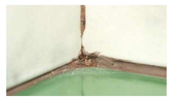
**1. A joint affected by mould** formation in a sanitary area must be repaired.
