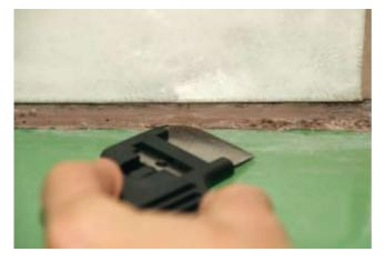
**2. Careful removal** of the affected sealant with a sharp blade.
