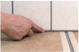
Backfilling the joint with OTTO PE backup foam rod in the appropriate size. The foam size must be chosen so that it requires a certain amount of pressure to insert it. Only then the joint is guaranteed to be filled out completely and the joint depth limited, too.
