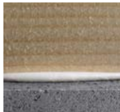
Wood on concrete
