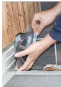
Adhesion of stainless steel to concrete bases
