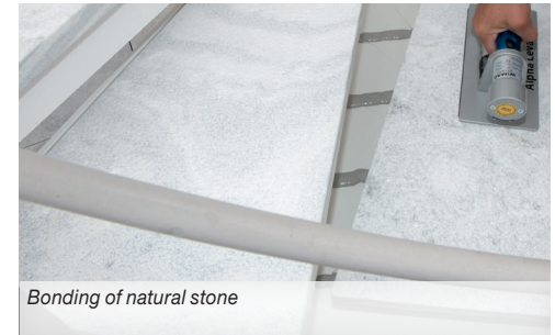
Facade plaster and metal – two materials come together
